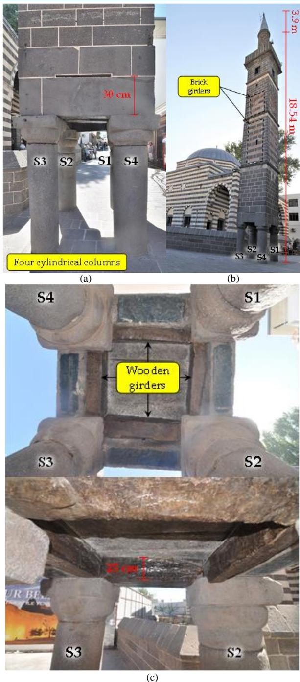
**Figure 3.** Photographic view of: (a) four cylindrical columns (west view), (b) brick girders (west and north views), and (c) wooden girders (bottom view)
